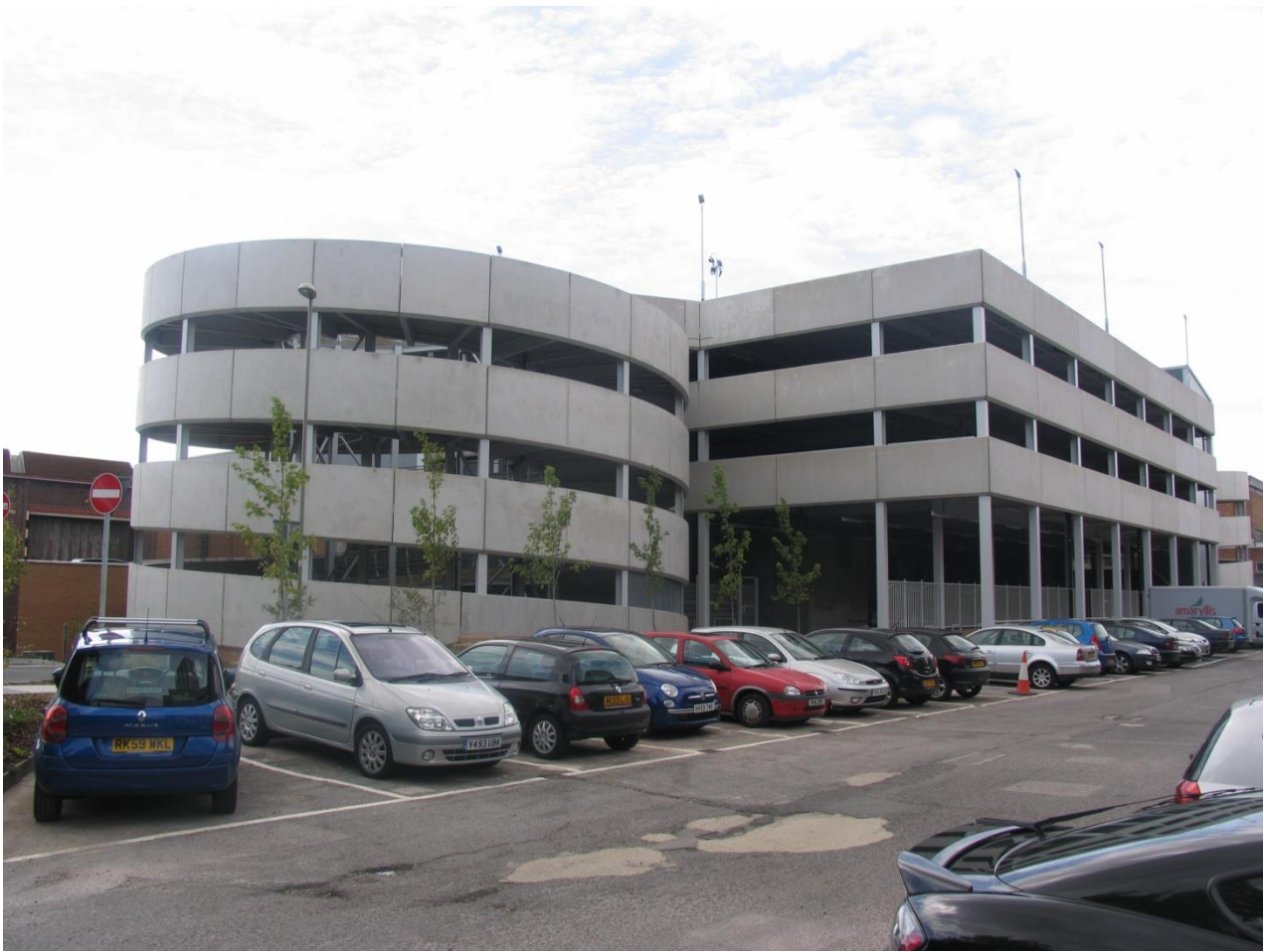
Fareham Shopping Centre Multi Storey car park
